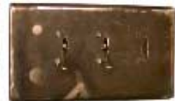
Air Switch Boxes
