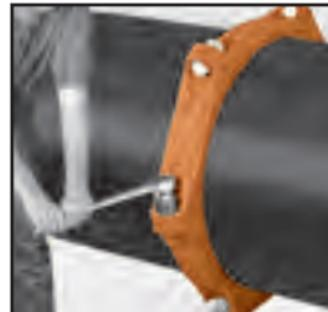
**7** Firmly torque each bolt. The specified minimum torque for each nut is 600 ft.-lbs. The specified maximum torque for each nut is 800 ft.-lbs.
