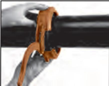
**4 Housings**—Put one half of the open coupling over the gasket as the coupling keys fit firmly into the grooves on each pipe end. Swing the other half of the coupling into position around the gasket and into the grooves.
