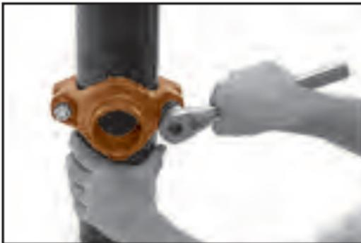
**5 Tighten nuts**—Alternately and evenly tighten the nuts to the specified bolt torque.
