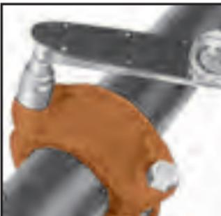
**6** Tighten the nuts alternately and uniformly until the required bolt torque is reached. See chart on previous page for bolt torque.
