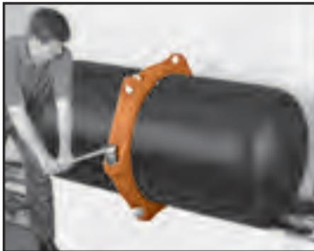
The instructions are based on pipe grooved in accordance with Gruvlok® grooving specifications. Check pipe ends for proper groove dimensions and to assure that the pipe ends are free of indentations and projections which would prevent proper sealing.
