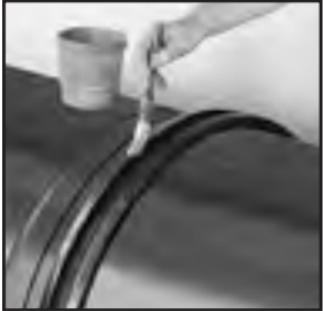
**3** Lubricate the gasket sealing lips. The use of Gruvlok lubricants ensures compatibility between the lubricant and the gasket.
