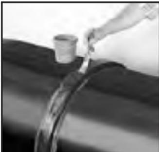
**5** Lubricate the exterior surface of the gasket. This helps prevent pinching of the gasket during assembly.
