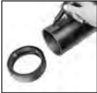
**2** Mark each pipe at a distance from the pipe end according to the pipe run size. See the chart.
