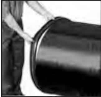
**2** Turn the gasket inside out and slide the gasket completely over one of the pipe ends. Turning the gasket inside out will reduce the stretching necessary to put the gasket into position. Ideally, approximately 75% of the pipe's gasket-sealing surface, (Dimension A) should be visible when the gasket is in proper position. This will aid in step 4.
