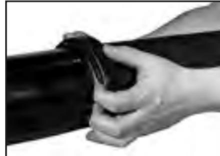
**3 Alignment—** After aligning the two pipe ends, pull the gasket into position centering it between the grooves on each pipe. Gasket should not extend into the groove on either pipe.
