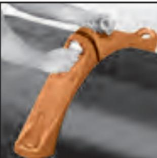
**6** Secure the housings about the pipes making sure the coupling keys are engaged in the pipe end grooves. Hint: For horizontal assembly, place housing segment on top of the pipe to support the weight of the housing segment. Secure the adjacent housing with an oval neck track bolt and heavy hex nut and then rotate the secured housings, again balancing the weight of the housings on the top of the pipe. Continue this procedure for all segments.
