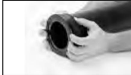
**3** Slip the gasket over one of the pipe ends. Make sure the gasket does not overhang the pipe end. Align the second pipe and while holding it in the butted position, slide the gasket back over the second pipe end. The gasket must be positioned on the gasket seat surface of the grooved steel pipe. Make sure the gasket does not overhang into the pipe groove.
