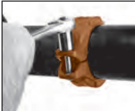
**5 Tighten Nuts—** Securely tighten nuts alternately and equally to the specified bolt torque, keeping the gaps at the bolt pads evenly spaced.
