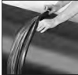
**4** Pull the two pipes into contact aligning the pipe ends.
